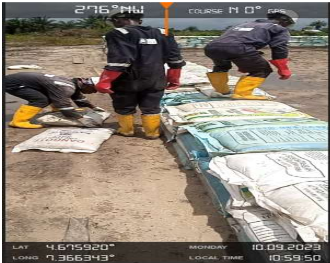
Plate 4: Stacking of Sandbags ongoing
