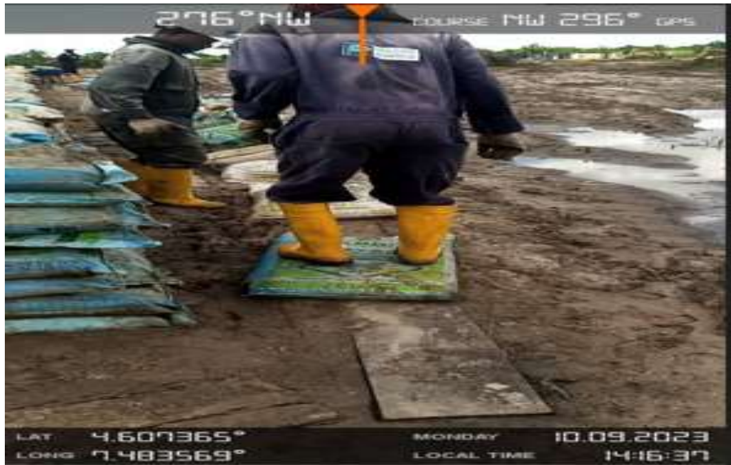
Plate 3: Laying of Sandbags
